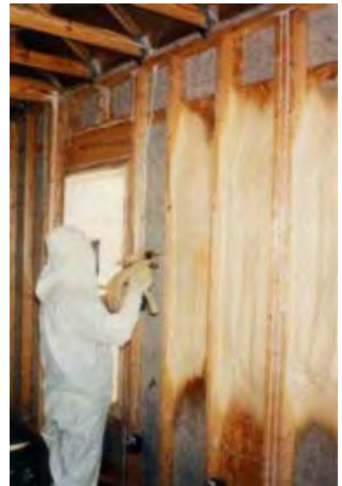
Application of NCFI spray insulation to stud wall cavity.
