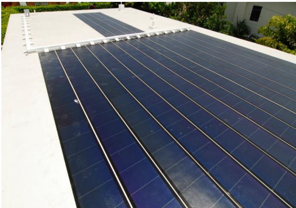
Figure 5 - Thin film, flexible PV panels adhered to roof surface
