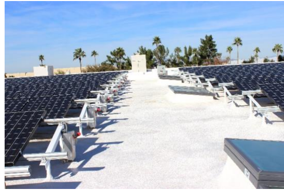
Figure 10 - Penetrating attachments with post/beam.
