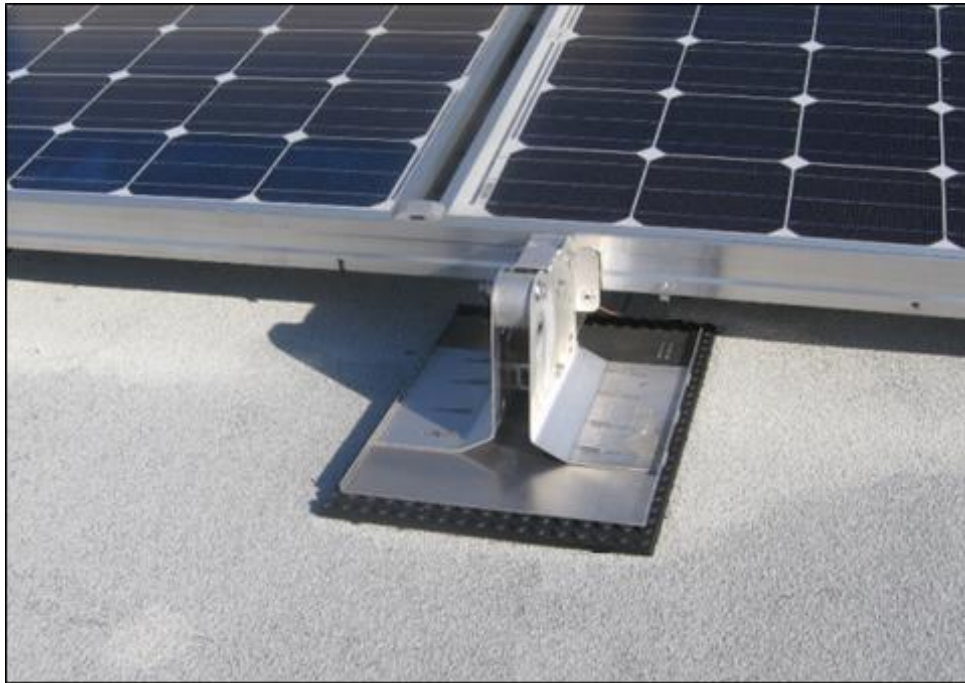
Figure 14 - Slip sheet under non-penetrating support of ballasted racking system.
