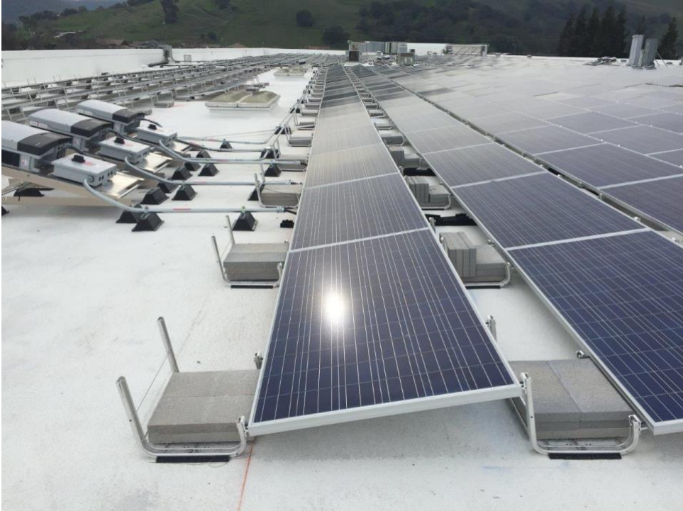
Figure 12 - Non-penetrating, ballasted system
