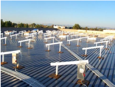
Figure 10 - Penetrating attachments with post/beam.
