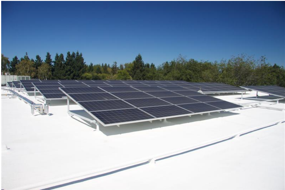
Figure 9 - Trusses between penetrating stand-offs.
