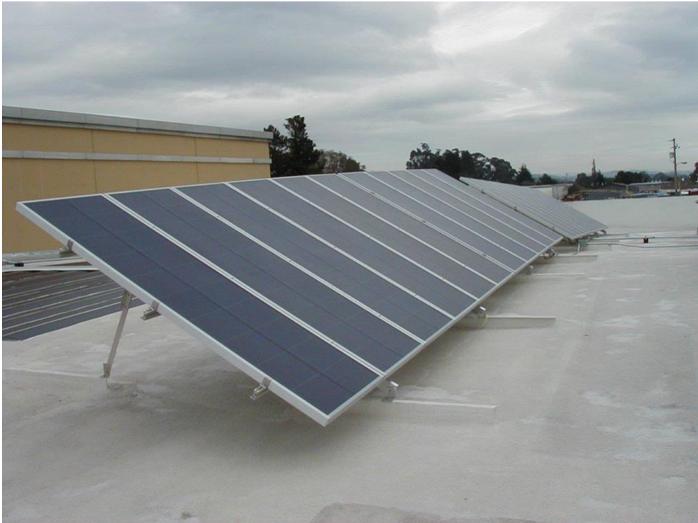
Figure 8 - Typical roof curb with truss supports.
