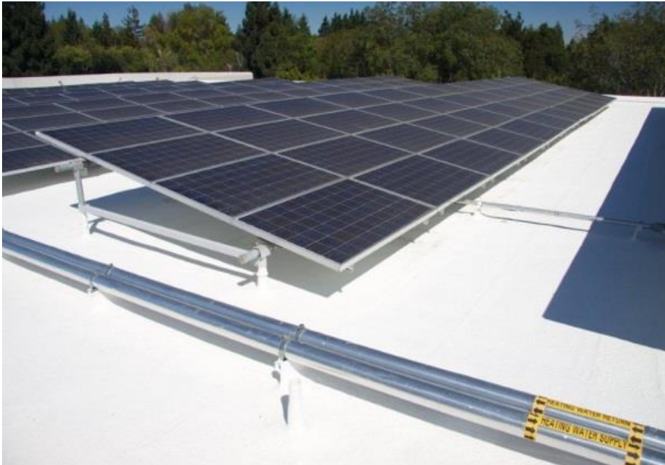
Figure 1 - Typical Penetrating Rack-Mounted PV System
