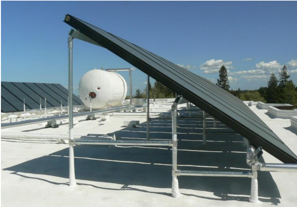
Figure 13 - Flashed stand-off attachment.
