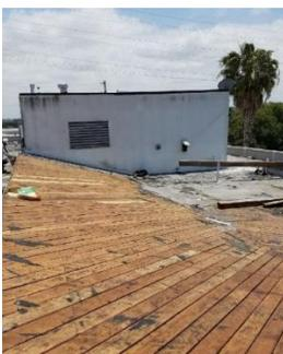
**Figure 1 - Roofing SPF Applied Directly to an OSB Wood Deck (top) and a Wood Plank Roof Deck Ready for Roofing SPF Application (bottom)**
