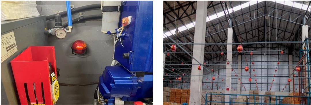
Figure 1 – Single and Multiple Fire Extinguishing Balls for Fire Suppression. (Single ball shown in an SPF rig)
