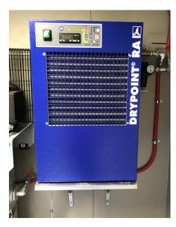
All Profoam Rigs come standard with a High Temperature Refrigerated Air Dryer
